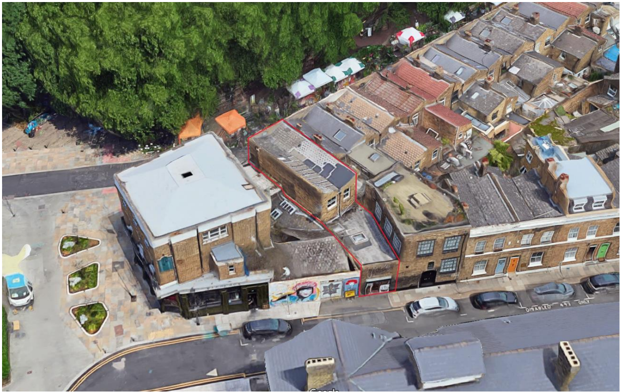
Aerial view of the site, from the south, looking at Wellington Row
