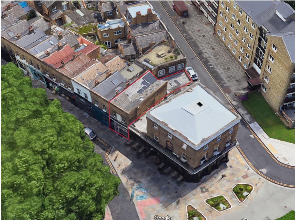
Arial view of the site, from the northwest, looking at Columbia Road
