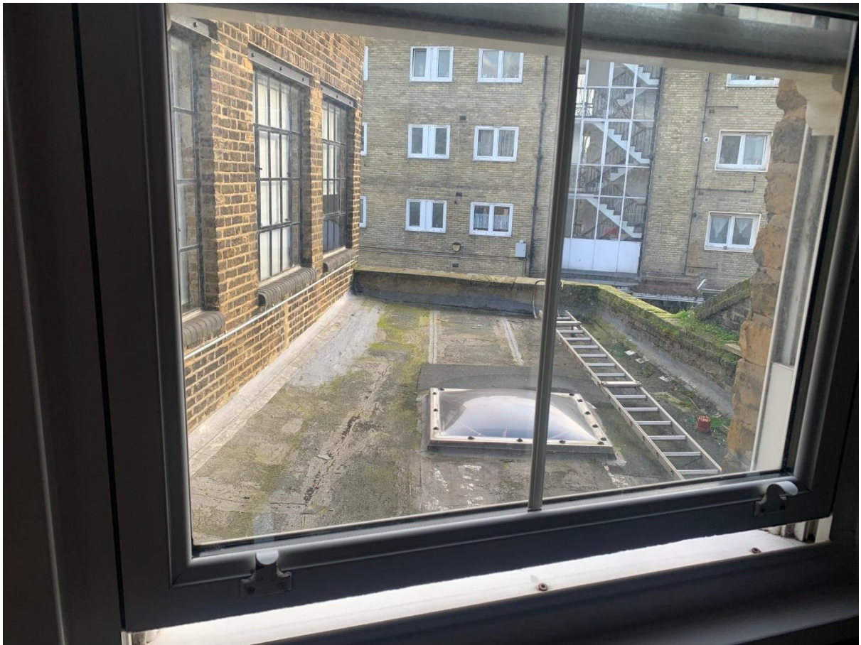
Rear extension view from upstairs flat window
