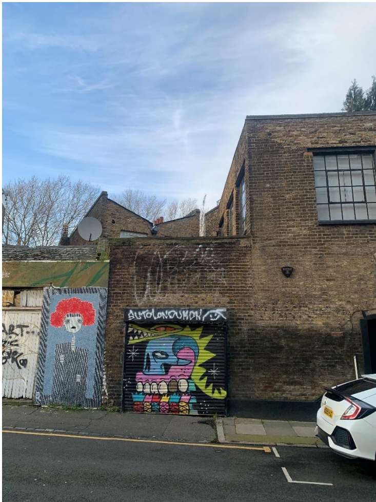
Rear of site, from Wellington Row
